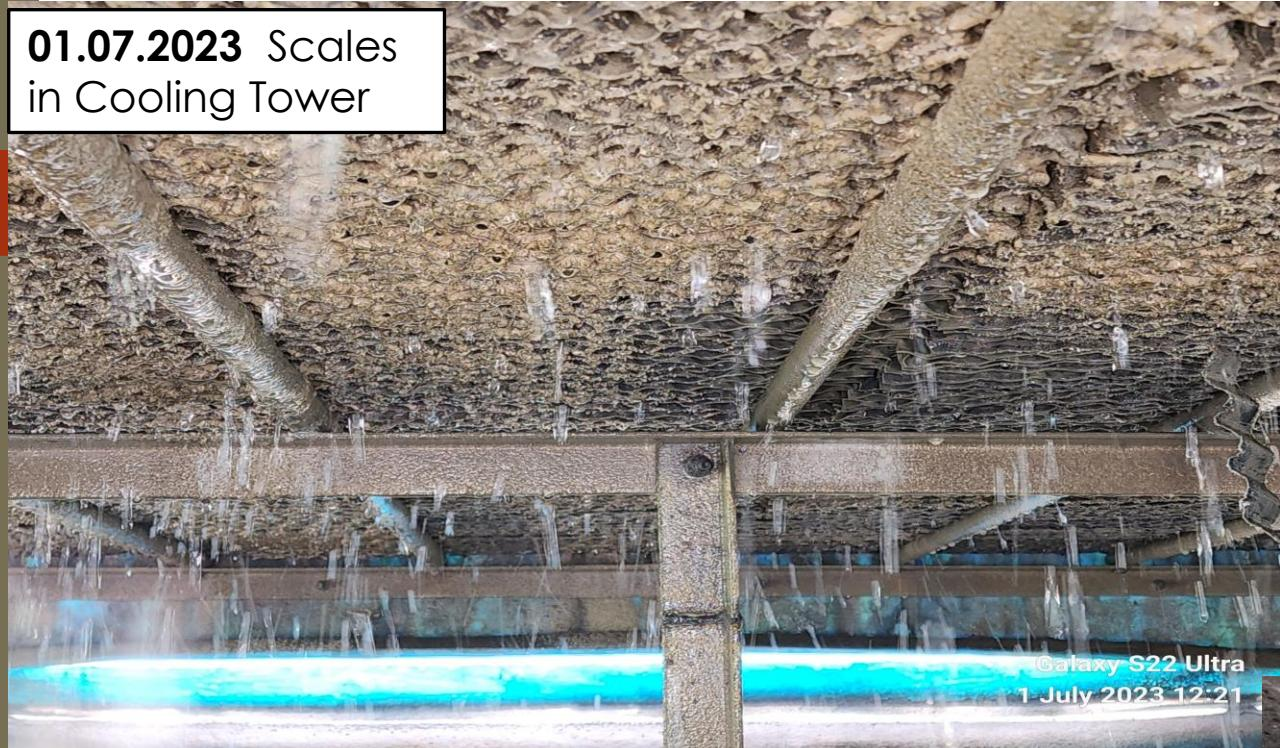
As on 01.07.2023, heavy scales were noticed on fills and Cooling Tower body.
